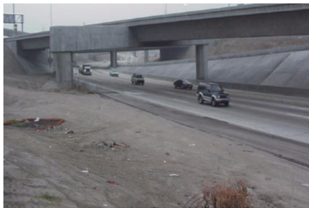
Figure 1. View of 91/5 highway over-crossing.
